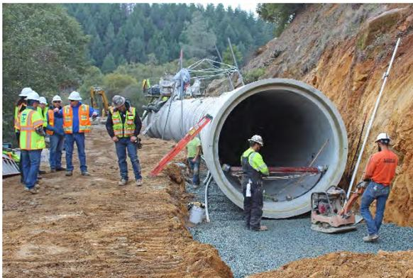
Work is on schedule to have water flowing through the new pressure pipe that is replacing the District’s Combie Phase 1 Canal.
