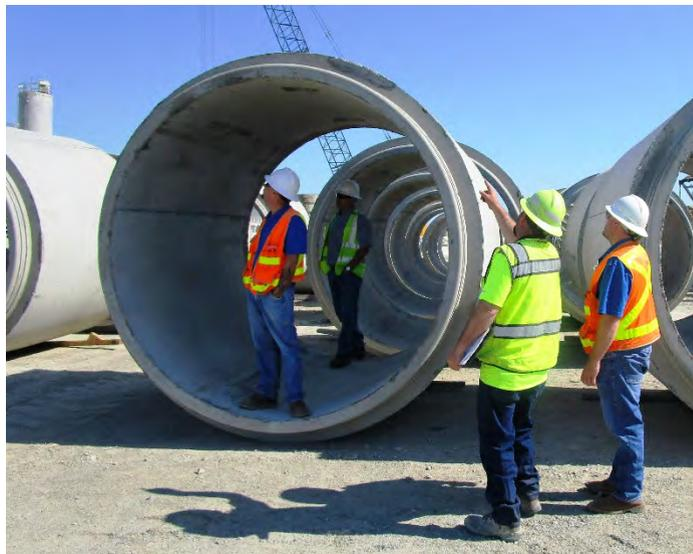
NID personnel inspect new pipe segments that will be used to replace the canal.
