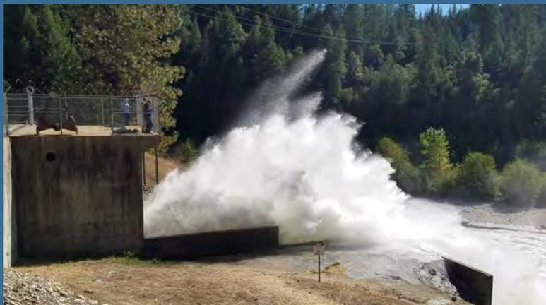
At the Chicago Park Powerhouse, hydroelectric experts survey testing of a full load rejection. The test included ramping up the powerhouse to its maximum generation and causing it to shut down in an emergency fashion.
