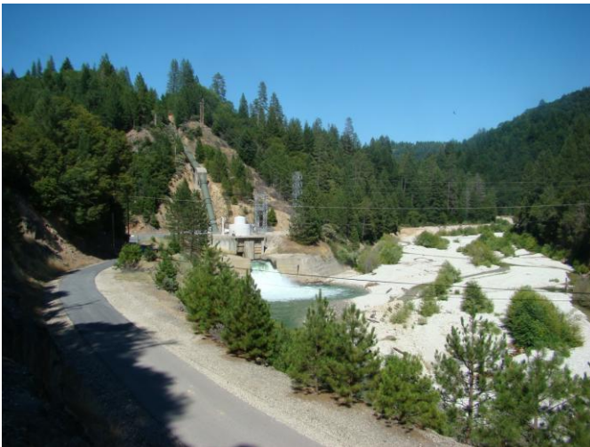
Chicago Park Powerhouse
