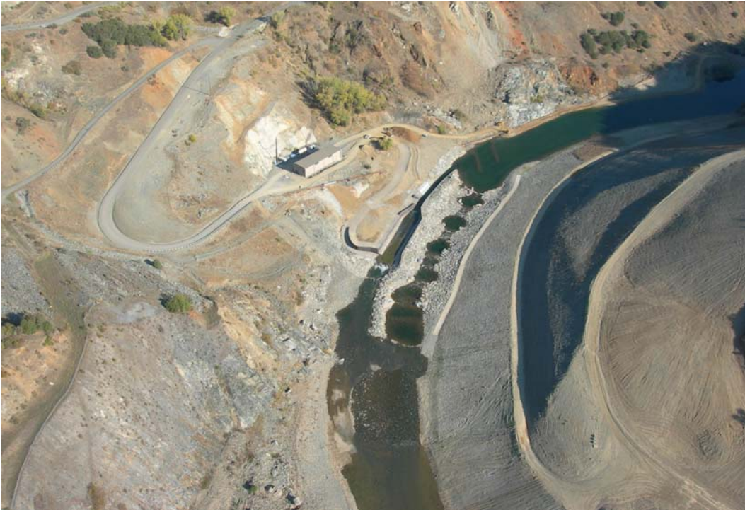
Figure 6.5.3-5. PCWA's American River Pump Station on the North Fork American River.
