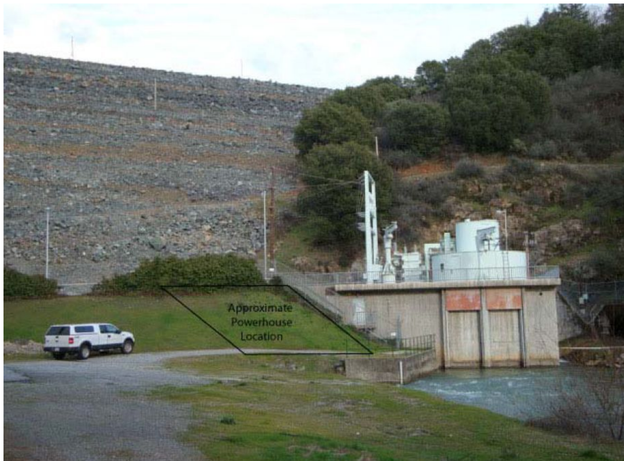
Figure 5.2.1-1. Approximate location of proposed Rollins No. 2 Powerhouse (existing Rollins Dam and Powerhouse are shown).
