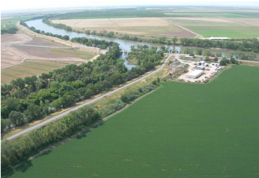
Figure 6.5.3-22. Cross Canal entering Sacramento River.
