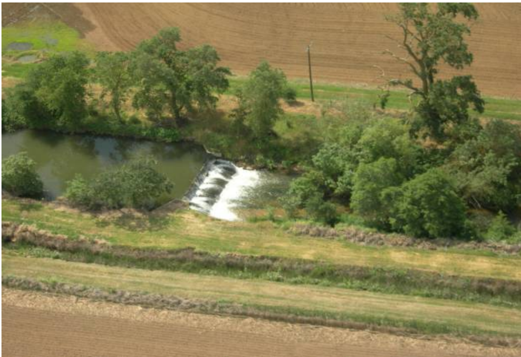
Figure 6.5.3-16. Unidentified diversion dam on Lower Auburn Ravine.
