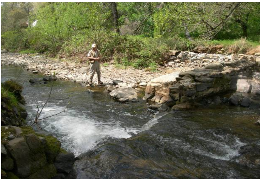
Figure 6.5.3-7. Private diversion dam located near RM 27.2 just below North Ravine. The diversion canal is located to the right of the person standing next to Auburn Ravine.
