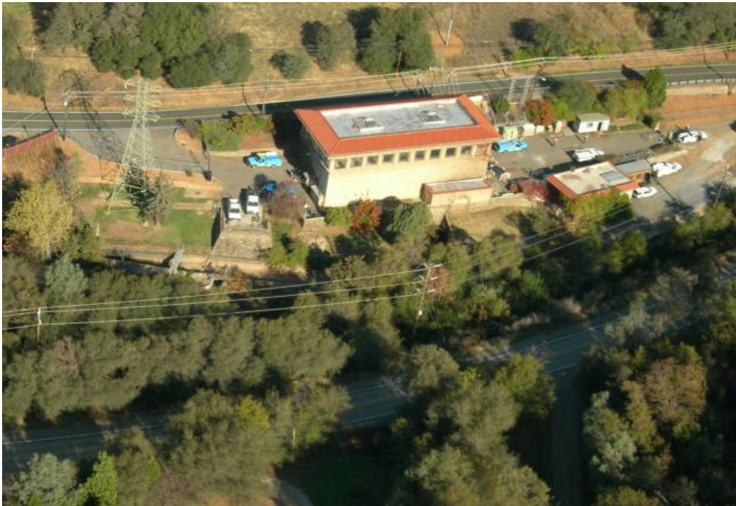
Figure 6.5.3-3. Aerial photograph of Wise Powerhouse and Wise Powerhouse No. 2, November 5, 2007.
