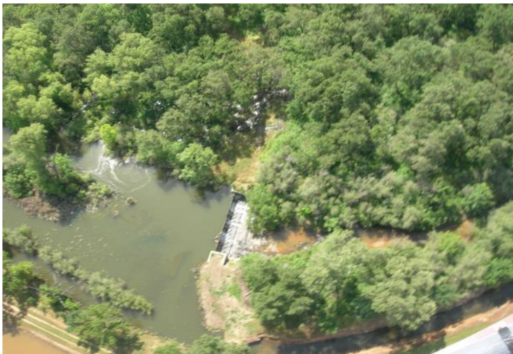
Figure 6.5.3-18. Unidentified diversion dam on Lower Auburn Ravine.
