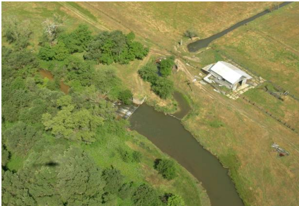
Figure 6.5.3-17. Unidentified diversion dam on Lower Auburn Ravine.
