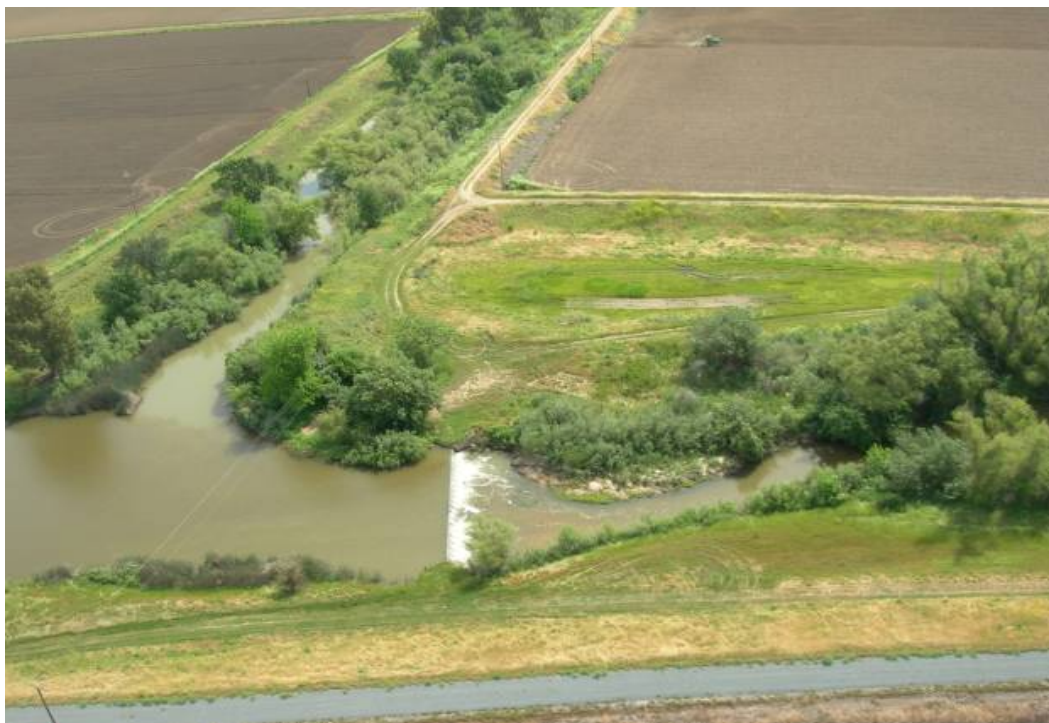
Figure 6.5.3-19. Auburn Ravine entering East Side Canal just above Coppin Dam. Auburn Ravine enters East Side Canal from the top of the photograph.
