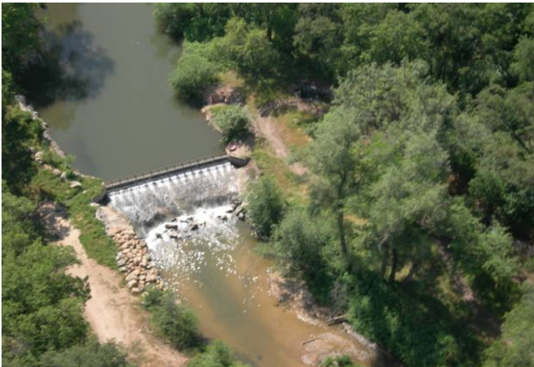
Figure 6.5.3-12. NID's Hemphill Diversion Dam at RM 17.5.
