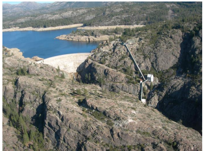
Lake Spaulding Dam and Powerhouses No. 1 and No. 2
