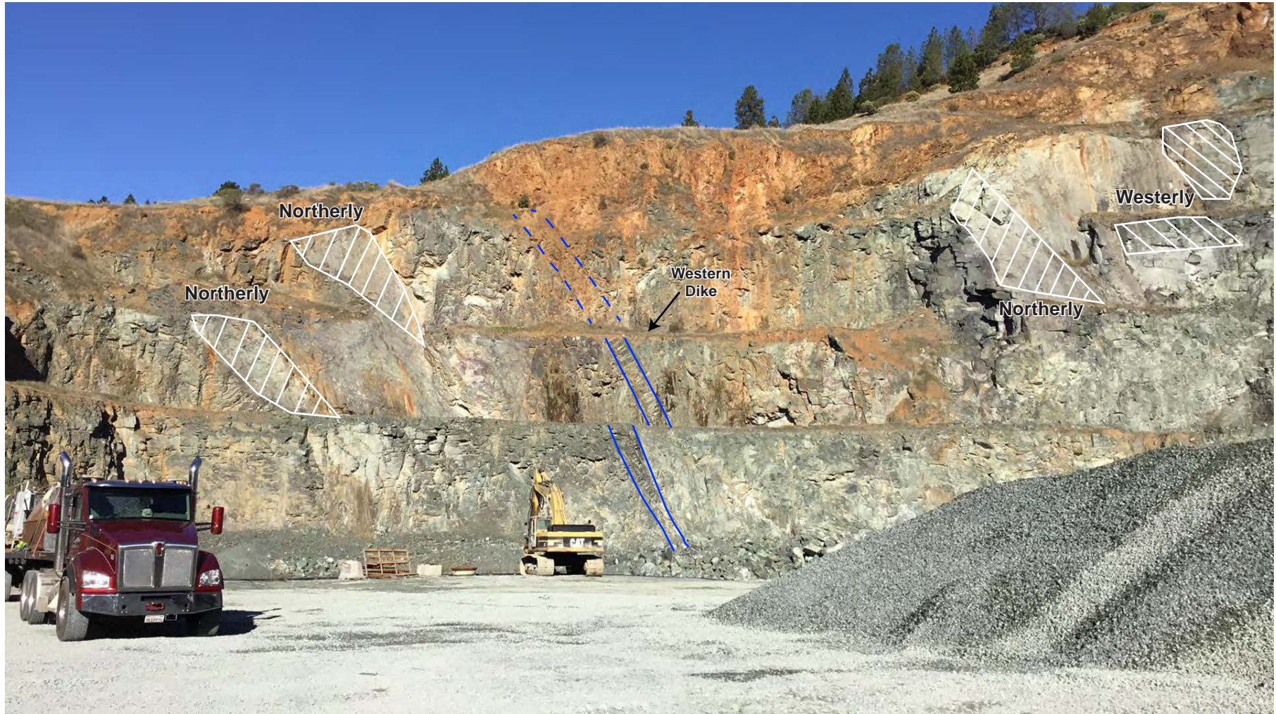
View to the northwest within Teichert Quarry showing the location of the western mafic dike, intersection of approximately north-south and east-west oriented joints, and large continuous rock faces along preferred jointing.
