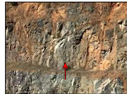
Ⓒ Intersection of N-S and E-W trending joints (approximate)
