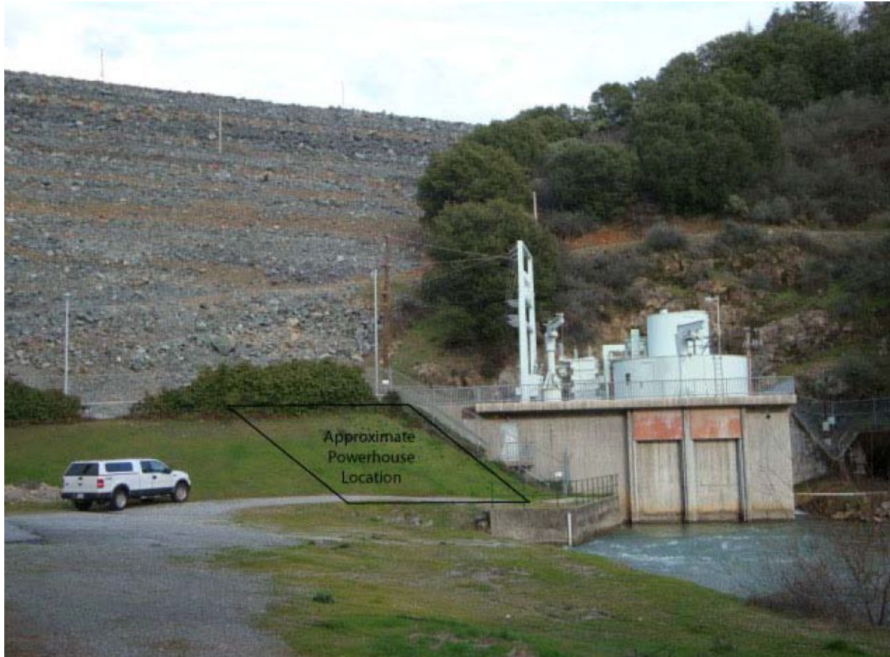
Figure 6.1-1. Anticipated location of proposed Rollins No. 2 Powerhouse (existing Rollins Dam and Powerhouse are shown).
