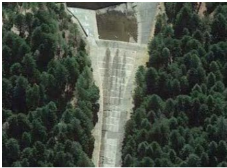
Scotts Flat Spillway
