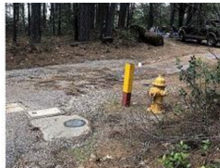
2684-2 Street view with fire hydrant
