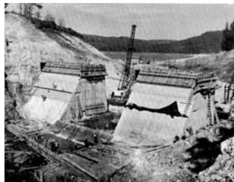
Building Scotts Flat Dam, 1964
