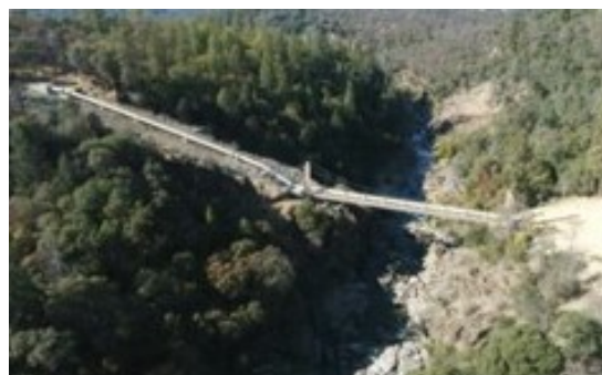
The aerial siphon crosses the Bear River.
