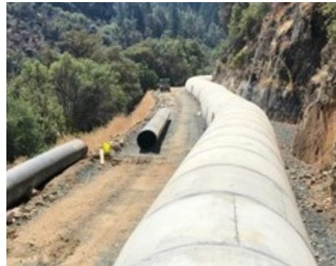
The Combie Phase I Pipeline stretches 1.7 miles.
