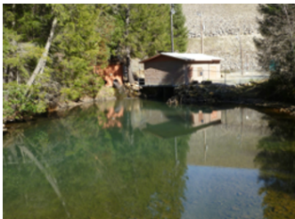
Scotts Flat Powerhouse
