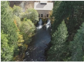
Deer Creek Powerhouse
