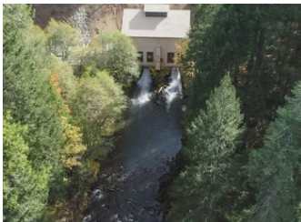
Deer Creek Powerhouse
