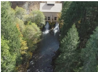
Deer Creek Powerhouse
