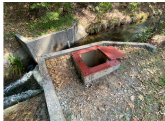
Lower Grass Valley Canal Head Gate/Gaging Station (Below)
