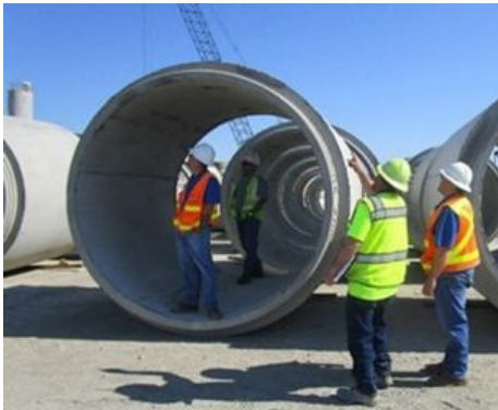
Inspectors look over the massive concrete pipe segments.
