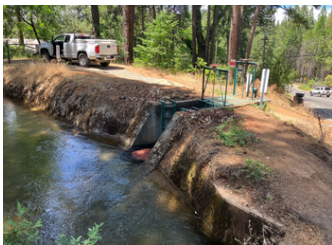
Lower Grass Valley Canal Head Gate
