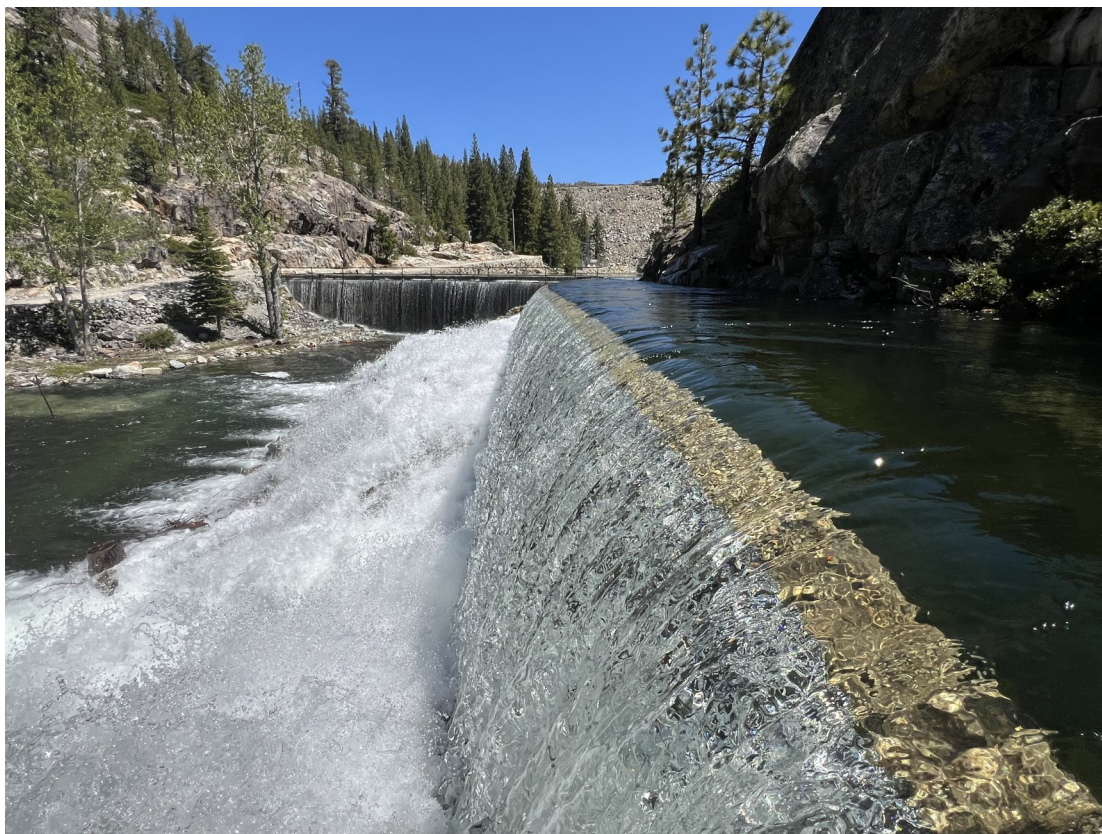
Snowmelt at the Canyon Creek Diversion Dam, Head of the Bowman-Spaulding Canal, and Bowman House. May 16, 2024
