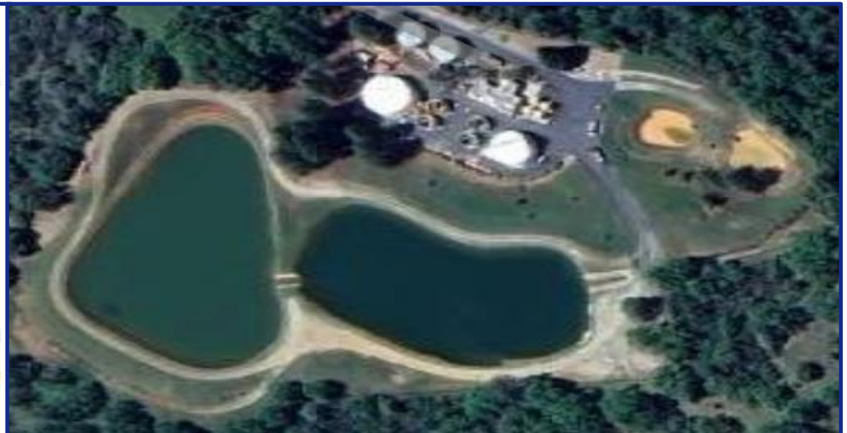
Lake Wildwood Water Treatment Plant
