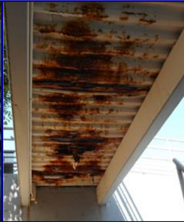
Underside of walkway to Operations entrance
