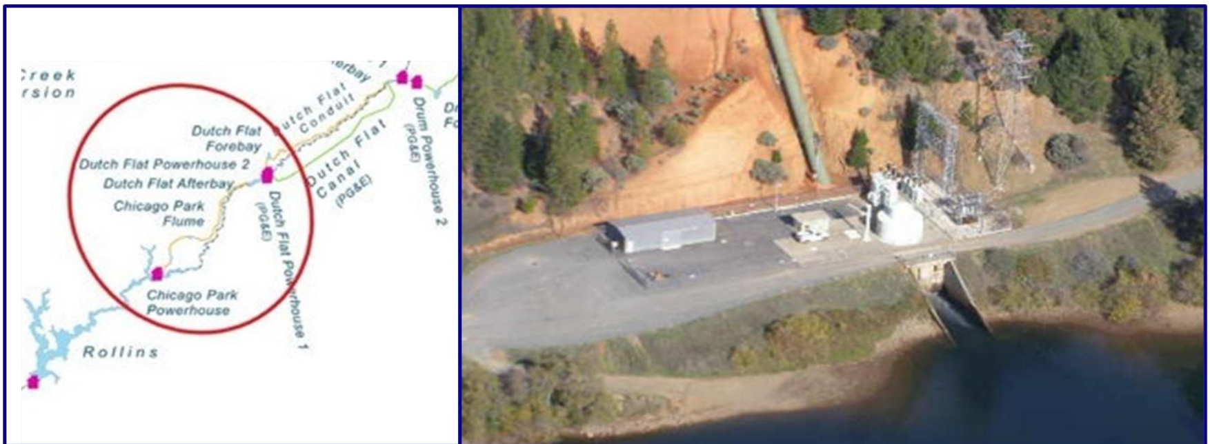
Dutch Flat #2 Powerhouse
