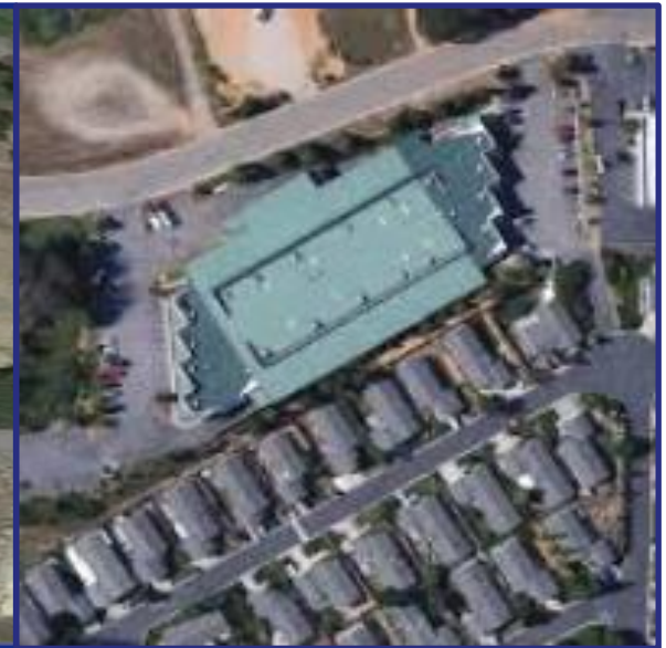
NID Hydro Electric Field Office Aerial View
