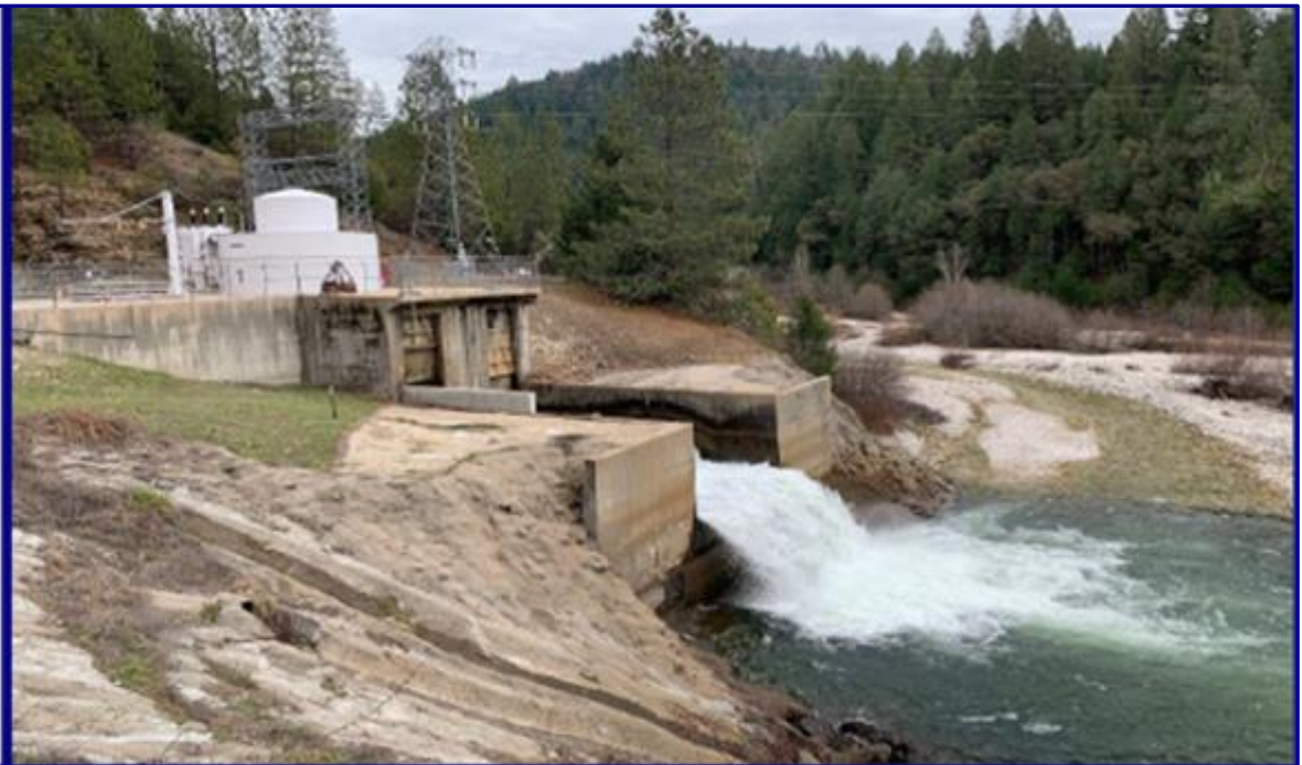
Chicago Park Powerhouse
