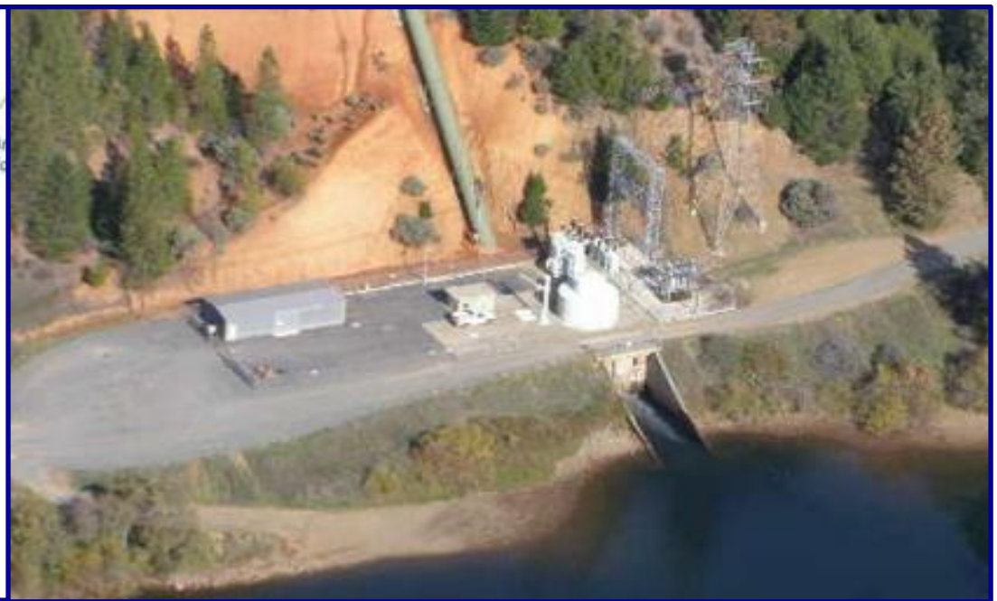
Dutch Flat #2 Powerhouse
