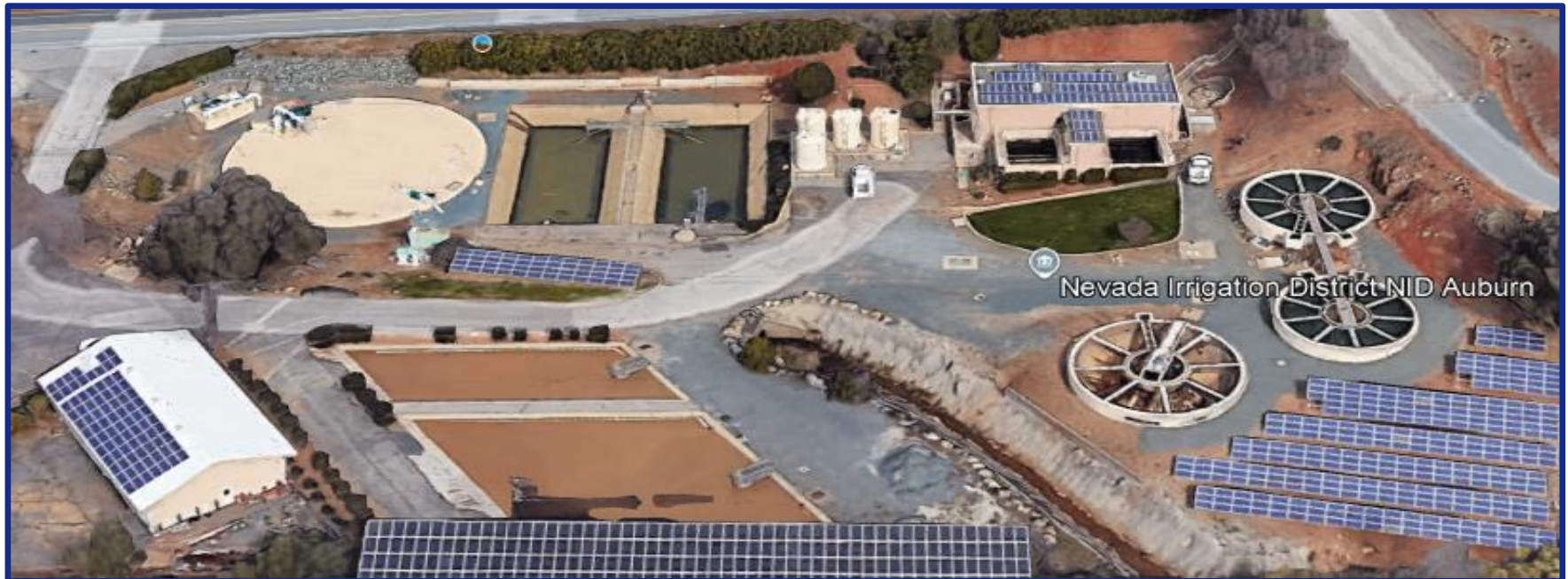
No. Auburn Water Treatment Plant
