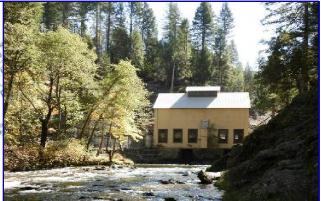
Deer Creek Powerhouse
