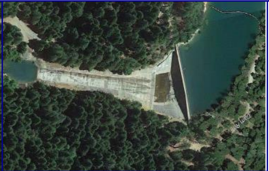
Scotts Flat Spillway
