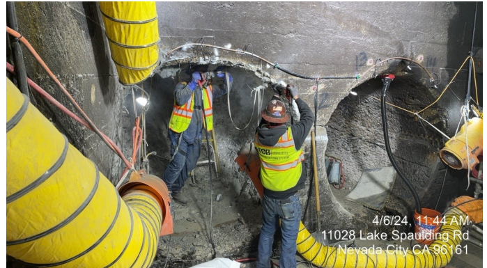
A PG&E crew makes repairs at Lake Spaulding..
