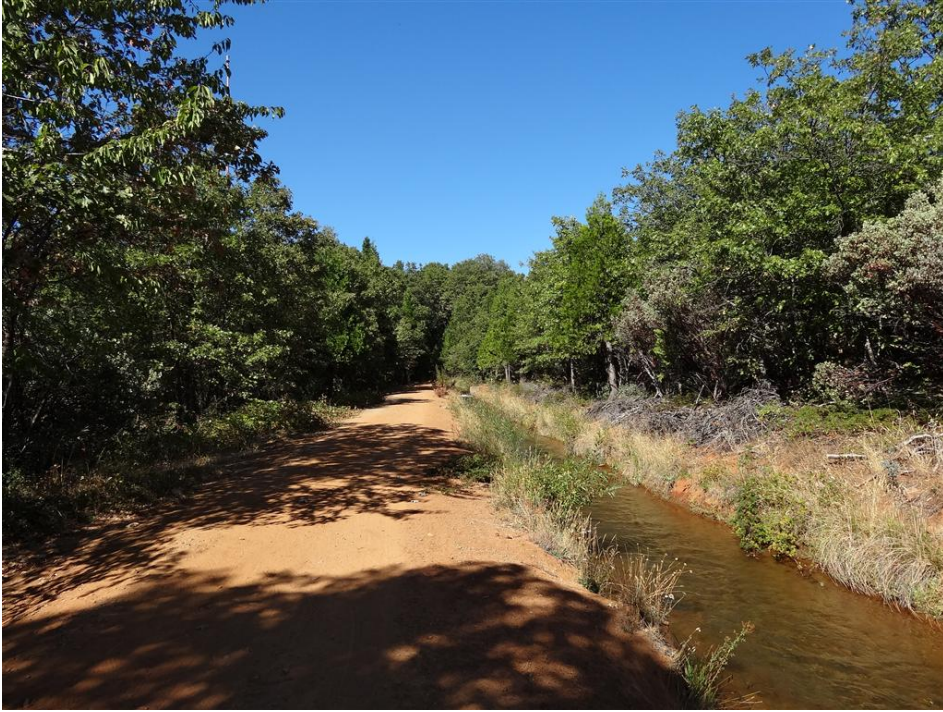
Looking north from southern most end of canal (before treatment plant)
