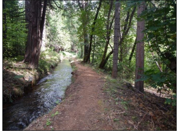
Lower Cascade Canal, study site 2. At study site access point, south aspect, facing downstream.
