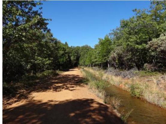
Photo 3: Lower Cascade Canal Mile 6 (as Identified in Figure 3)
