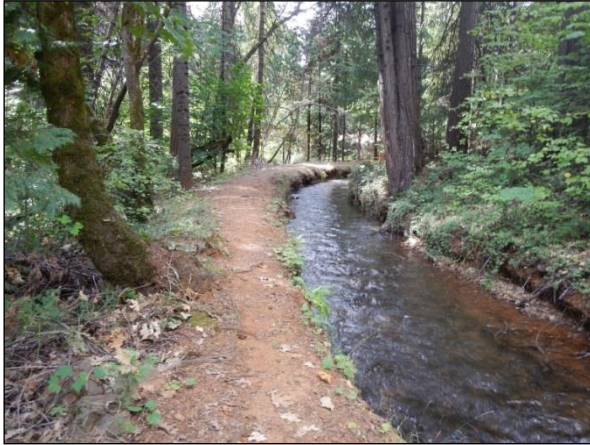
Lower Cascade Canal, study site 2. At study site access point, northwest aspect, facing upstream.
