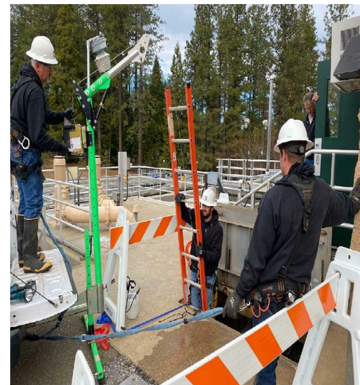
Confined space entry E. George valve inspection
