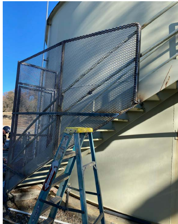
Insurance safety inspection completion of the encasement on the Lake of the Pines water treatment tank
