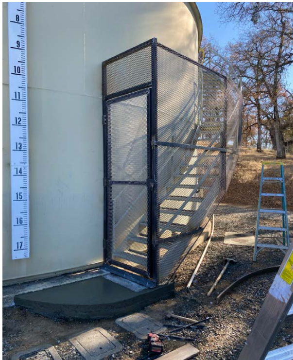
Insurance safety inspection completion of the encasement on the Lake of the Pines water treatment tank
