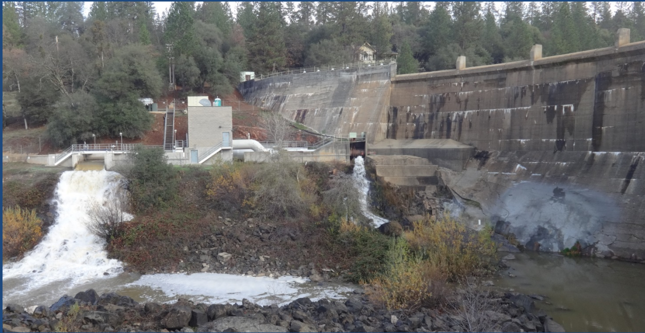
Combie Right Abutment
