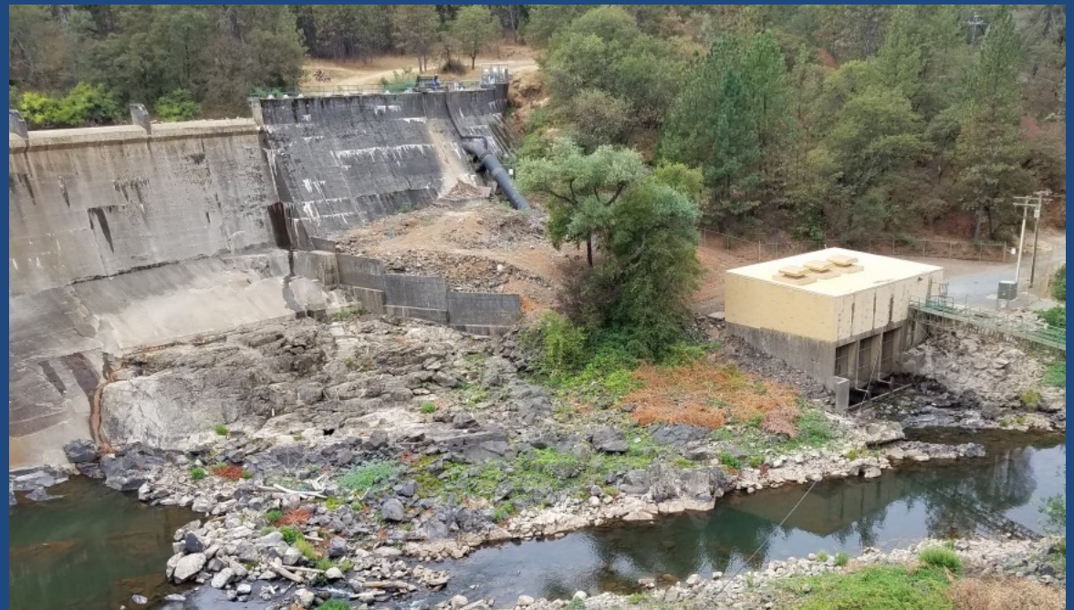
Combie Left Abutment
