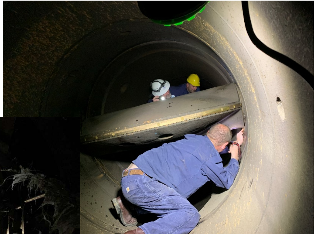
Inspection of Turbine Shutoff Valve at Dutch Flat #2 Powerhouse
