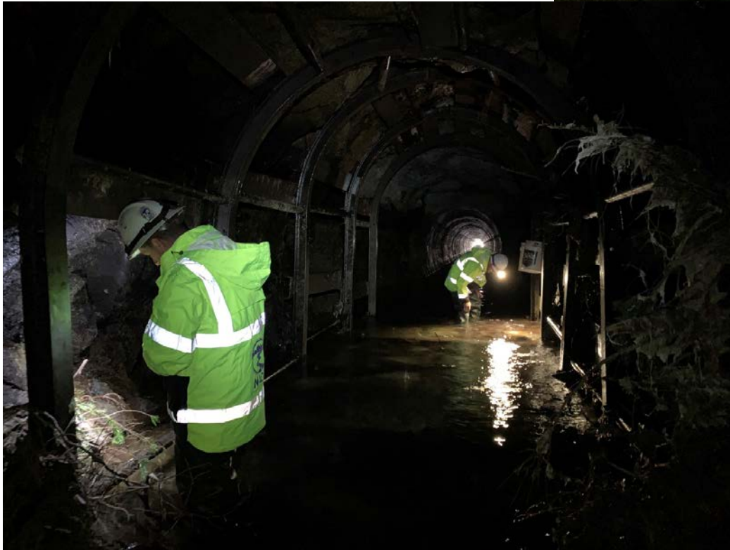
Clear Creek Tunnel Improvements
