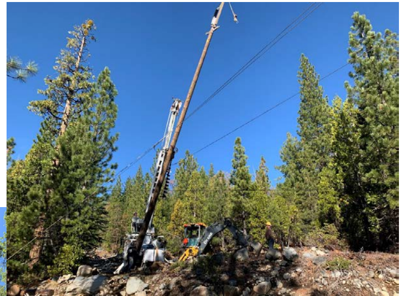
Bowman Transmission Line Pole Replacement
