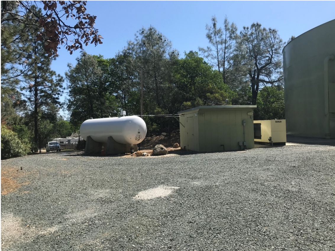
Existing pump station building, white pressure tank, generator and storage tank, northeast view
