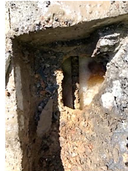
Emergency – Repaired/banded service line on Alta Vista Avenue (E. George System)
