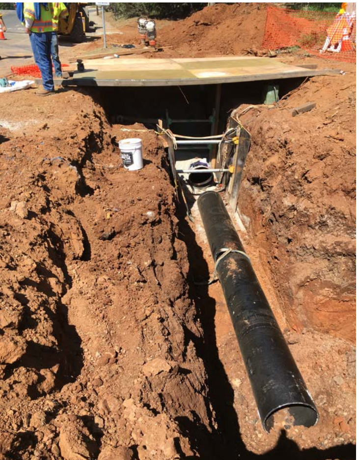
Ridge Road-Transmission Main Improvement
