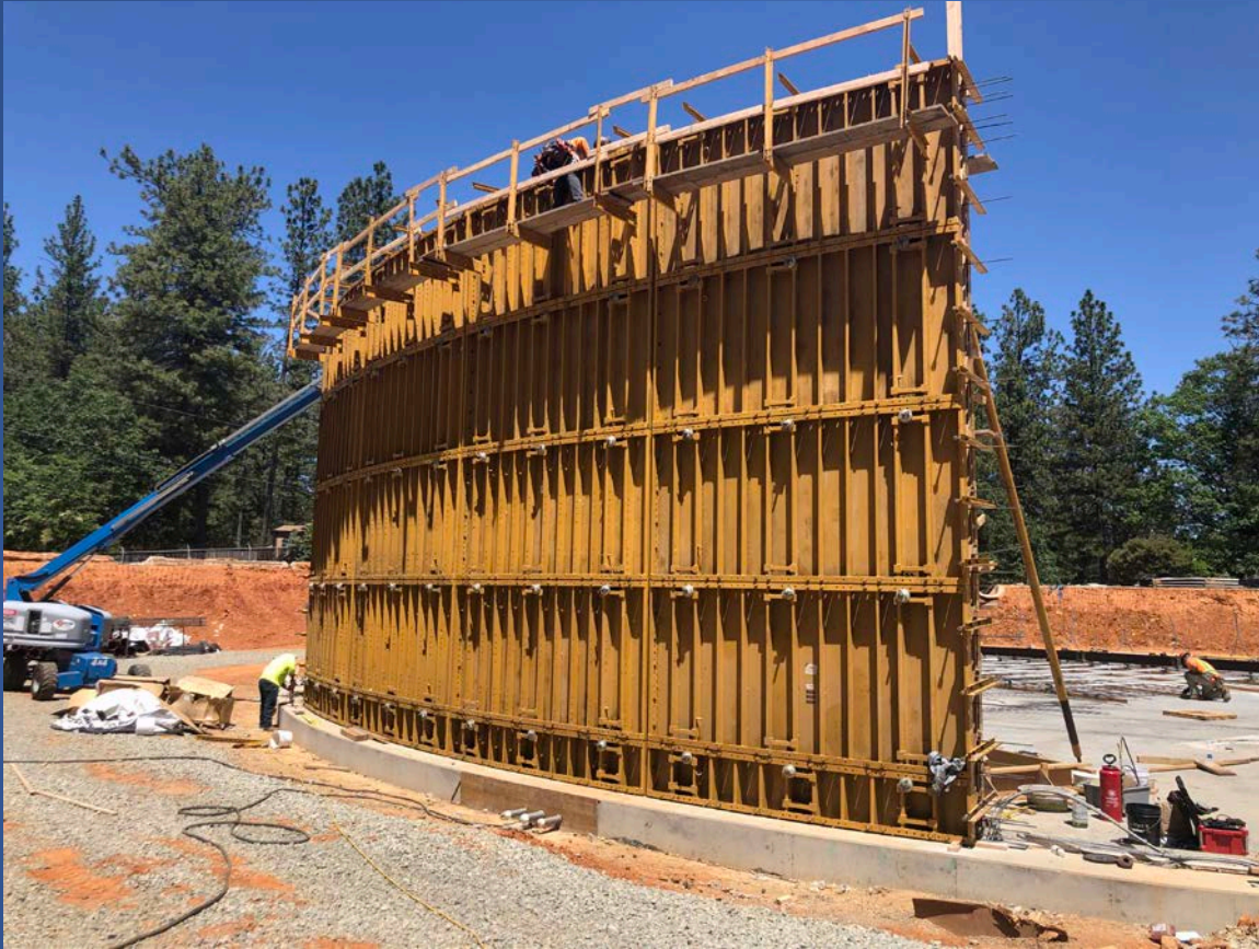
First wall of tank being poured
