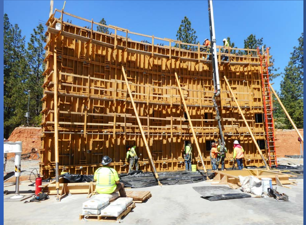
First wall of tank being poured
