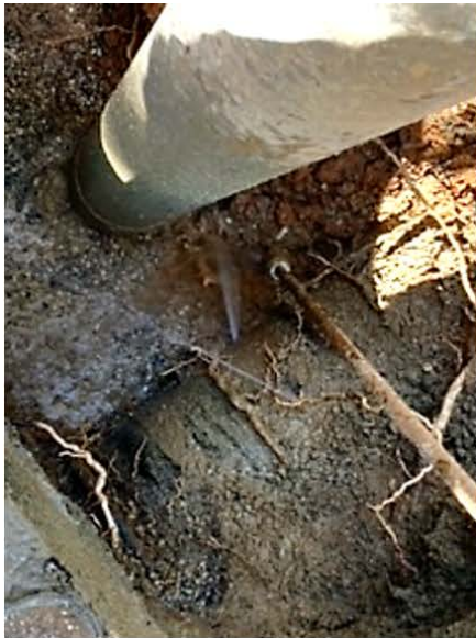
Emergency – Repaired 18' main line on Durbrow Road (E. George System).
