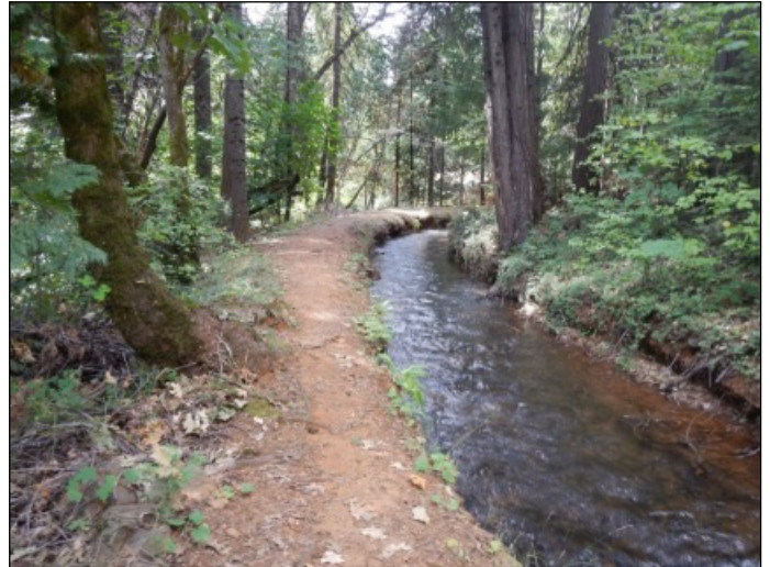
Photograph 6: 2013: LCC Site 2. Southwest facing aspect.
