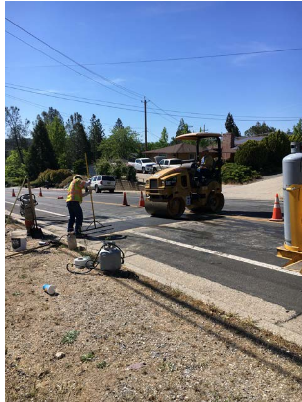
Patch paving-Huges Road after a leak
