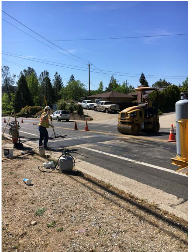
Patch paving-Huges Road after a leak
