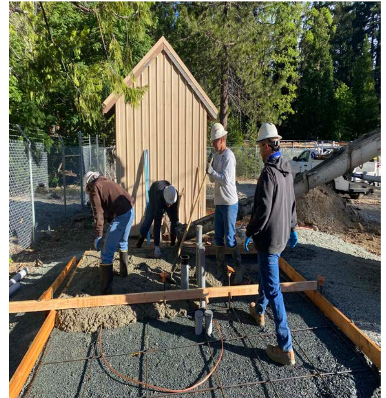
Bear Valley Yard-new foundation pad for new electrical panel
