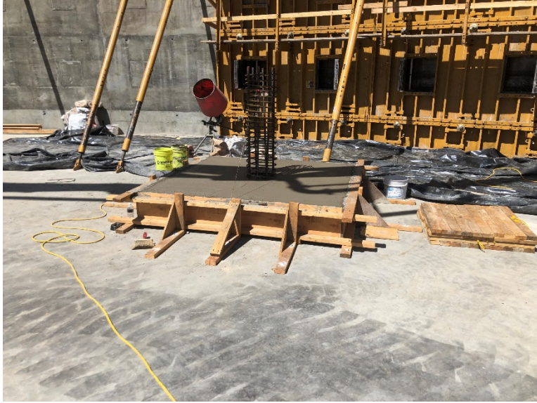
Alta Sierra Tank Site Construction
