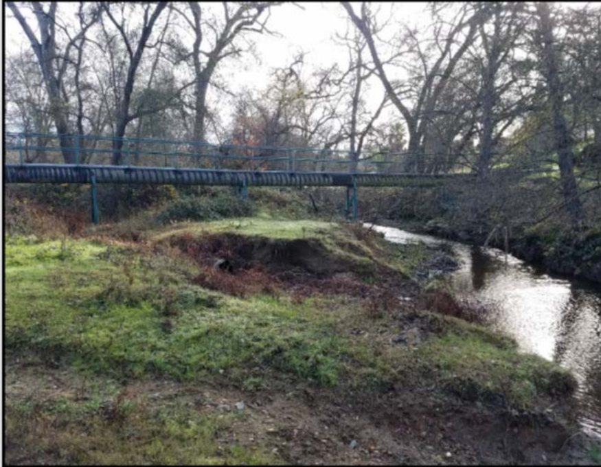
Photo 1: Standing on north bank of Doty Ravine, just below confluence of Doty Ravine and Sailors Ravine facing east.
