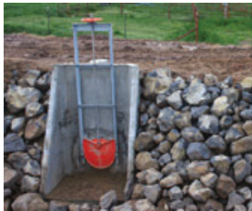
Remove existing manual gate and...
