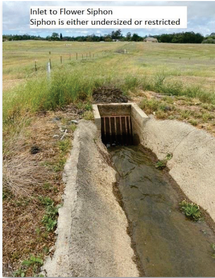
Lincoln Canal near Monument Pl Canal undersized
